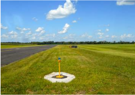
TAXIWAY LIGHTING REPLACEMENT Mankato Regional Airport (MKT), Mankato, MN
