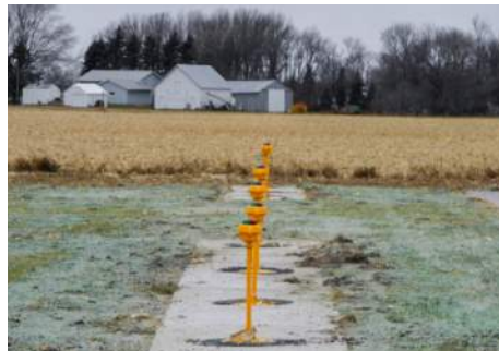
RUNWAY LIGHTING REPLACEMENT St. James Municipal Airport (JYG), St. James, MN
