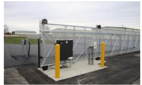
SECURITY FENCE IMPROVEMENTS Mankato Regional Airport (MKT), Mankato, MN
