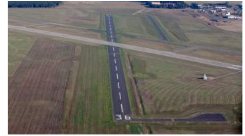
RUNWAY 18/36 PAVING AND LIGHTING Park Rapids Municipal Airport (PKD), Park Rapids, MN
