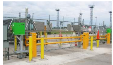
PERIMETER FENCE SECURITY IMPROVEMENTS Minneapolis-St. Paul International Airport (MSP), MN
