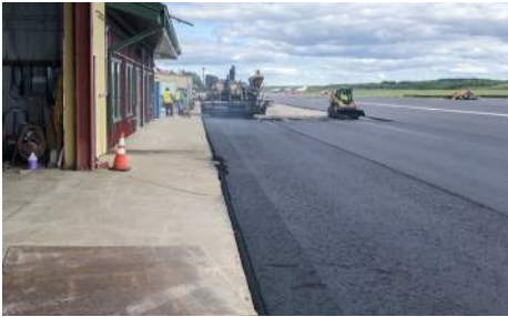
2018 PAVEMENT REHABILITATION Ely Municipal Airport (ELO), Ely, MN
