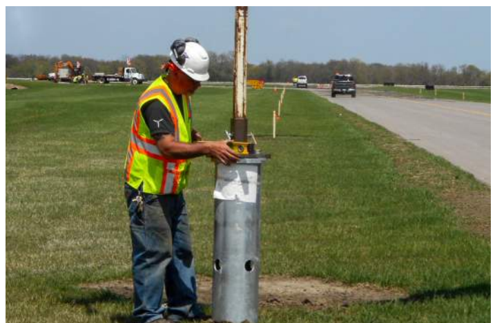
Mankato Taxiway Lighting Replacement
